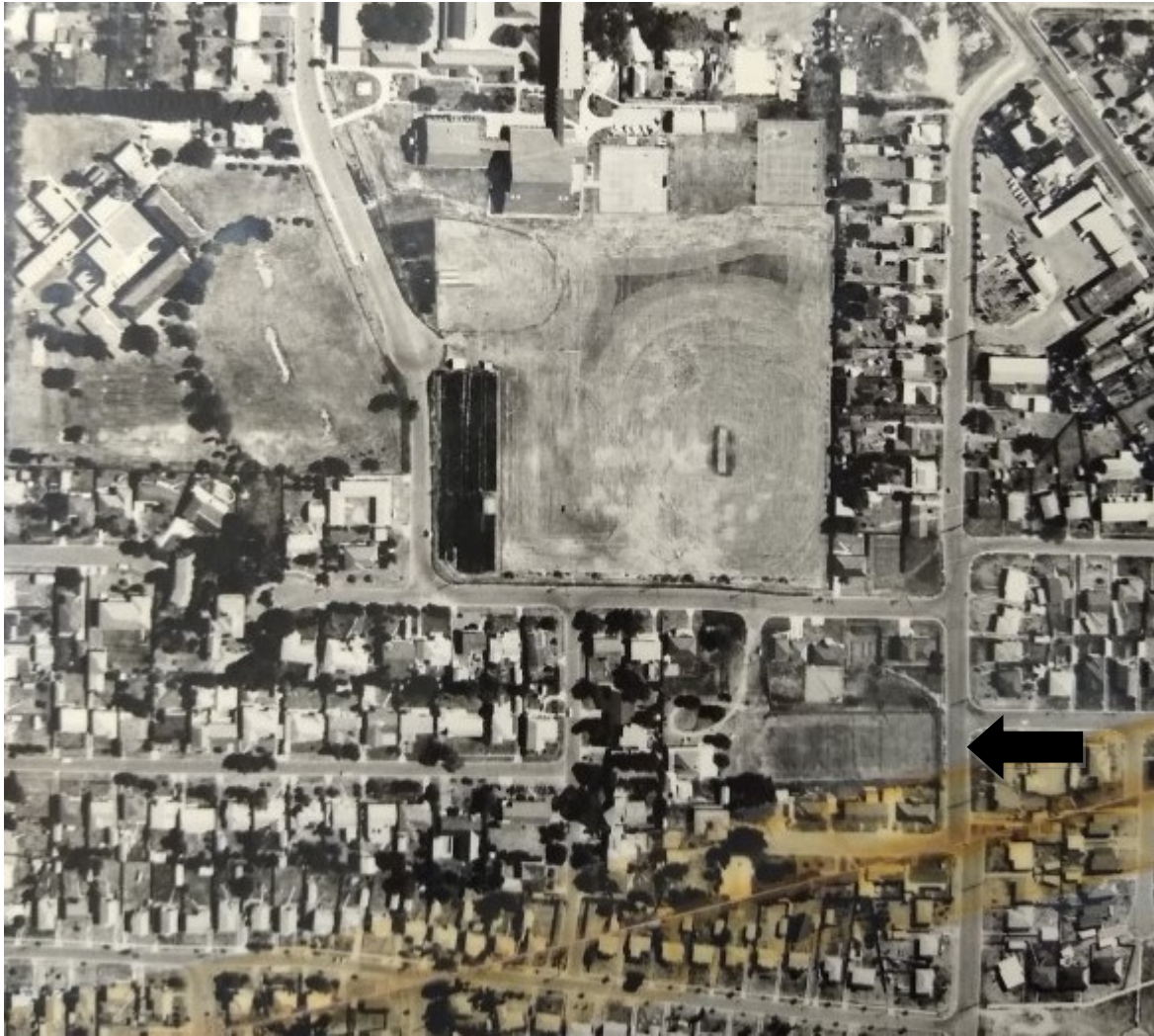
Figure 2.5: 1977 aerial photograph showing the club house and tennis courts (arrow) soon after the subdivision. Comparison to figure 2.4 shows the rapid infill of the former estates of Pelerin, Flowerbank and Townhead with housing, surrounding the Country Club. The Singleton High School and King Street Public School sit to the north of the site. The circular driveway is clear running from Edinburgh Avenue to the front of the club house (Source: Singleton Local Studies Archive Collection)
